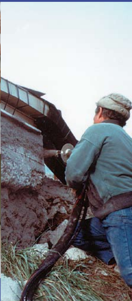
Remove spalled concrete from deteriorating structure.
